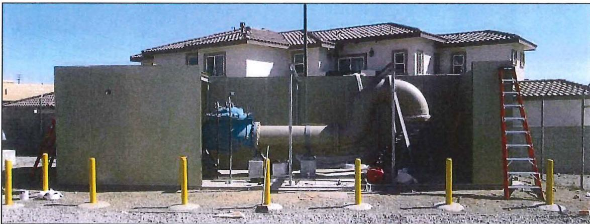
Completed installation of the south, east/west walls, and a third of north wall with roofing
